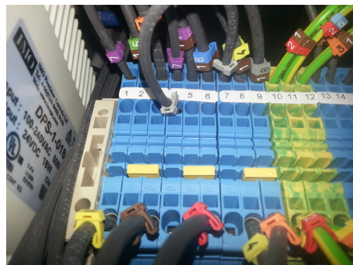
Delta Configuration: Jumpers across 2-3; 5-6; 8-9
